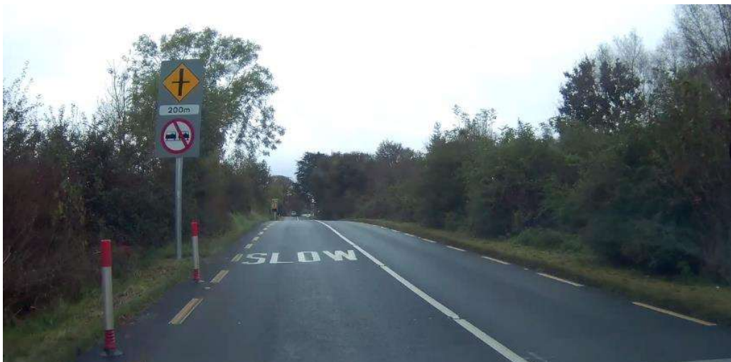
Figure 3-8 N3 north of Virginia travelling southbound on approach to local road cross-roads
