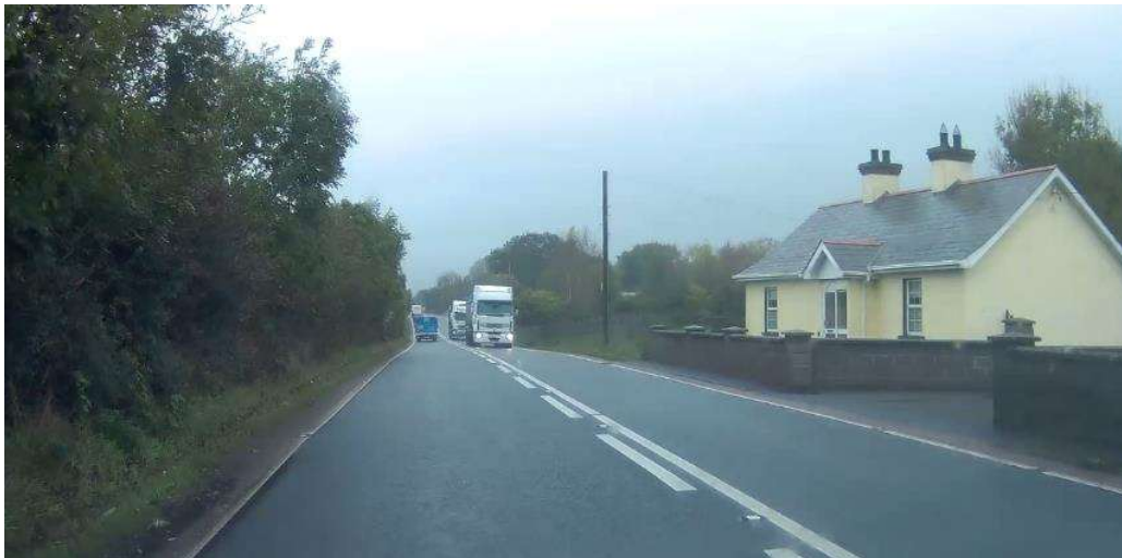
Figure 3-4 N3 south of Virginia travelling northbound
