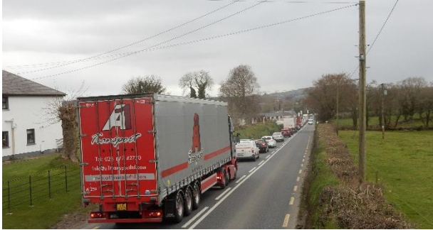
Plate 2-15 - Existing Traffic Queues along N3 Northbound towards Virginia Town. (≈3km from town at Burrenrea)
