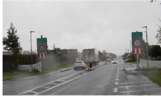
Plate 2-4 - Existing N3 in Maghera
