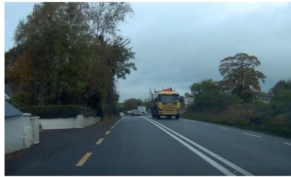
Plate 2-6 - Existing N3 between Maghera and Virginia (constrained cross section and roadside hazards)
