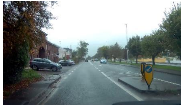
Plate 2-12 - Existing N3 within Virginia (north of town centre)
