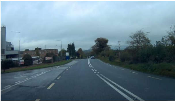
Plate 2-5 - Existing N3 between Maghera and Virginia (at HD15 site at Burrenrea, in vicinity of Glanbia Ingredients Ireland)
