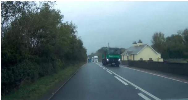
Plate 2-7 - Existing N3 between Maghera and Virginia (constrained cross section and roadside hazards)
