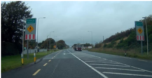
Plate 2-1 - Existing N3 between Derver and Maghera (Whitegate village gateway)
