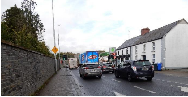
Plate 2-9 - Existing N3 within Virginia Town (R178 to Bailieborough traffic signals)
