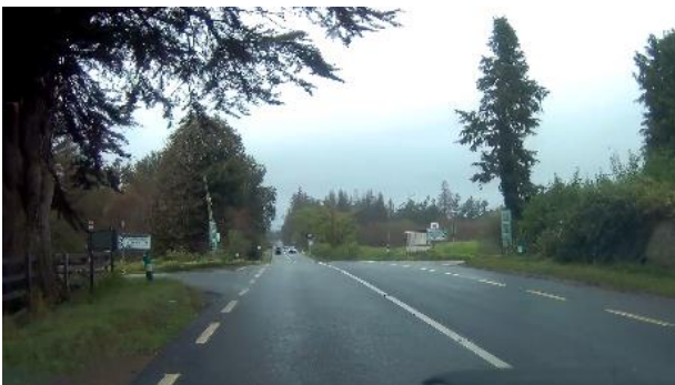
Plate 2-13 - Existing N3 north of Virginia (HD15 site at Murmod Cross)
